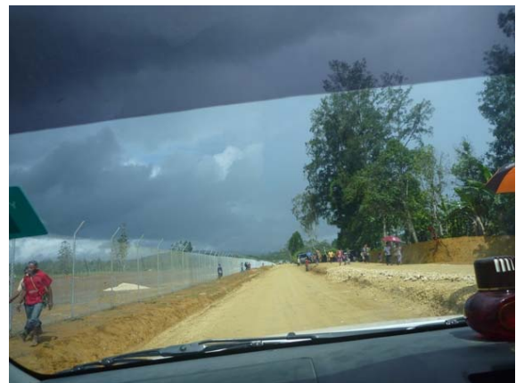
New airport being constructed at Komo in Southern Highlands
