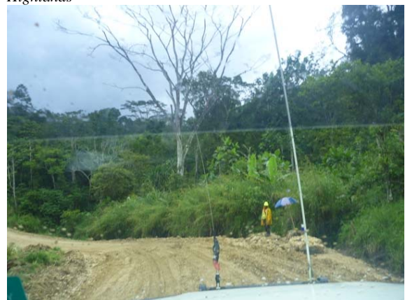
New road under construction in Komo and employment for local people
